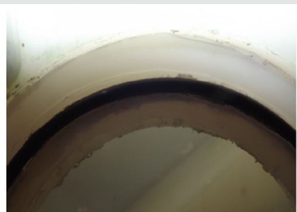
Figure 16: Valve opening: sealing with O-ring groove.
