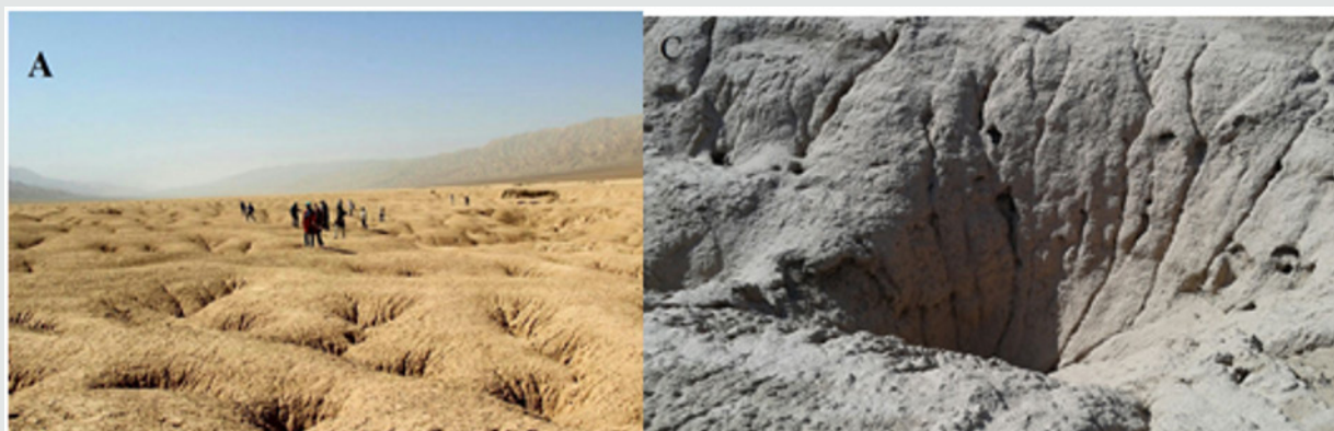
Figure 3: Site A with moderate piping and Site C with big depression.
