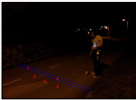
Figure 3: Locating Leakage Source of Underground Water Pipeline.
