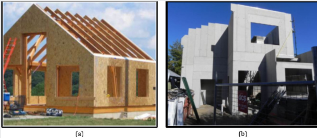
Figure 1: (a) SIP house with OSB skin [8]; (b) SIP house with fiber cement skin [8].
