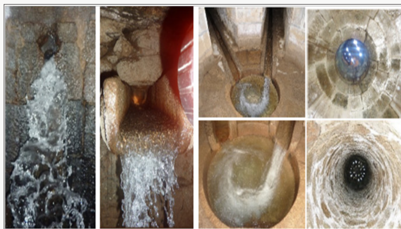
Figure 13: Water treatment processes performed inside the "chapels" (aeration, gas transfer, iron and manganese removal, sedimentation).
