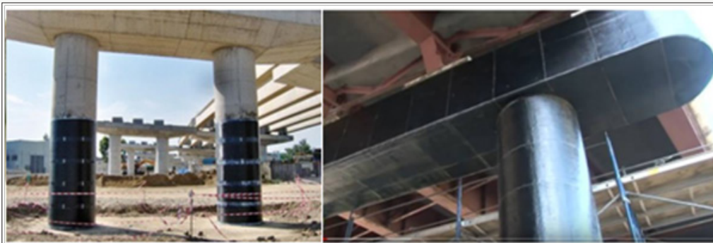
Figure 2: CFRP wrapped bridge columns and bent.
