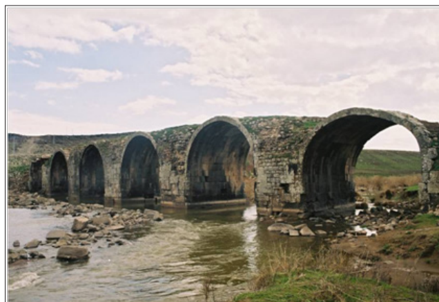
Figure 1: View of Karakopru direction from downstream.
