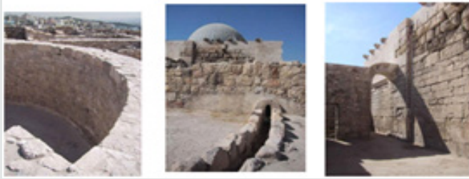
Figure 8: water harvesting in the audience hall, a) Down pipe collecting rainwater from roof, b) canals directed water to the cistern, c) View of cistern that functions as main water storage area.
