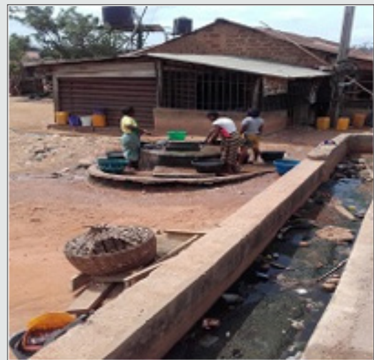
Figure 2(b): This shows a water channel being trashed with both solid and semi solid waste.
