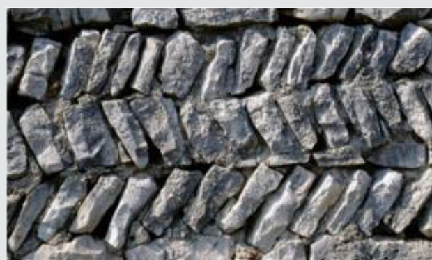
Figure 3: Side walls of the St Barbara Church built in the "fishbone" style (Photo by N. Fazinić).
