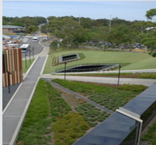
Figure 2: Part of Macquarie University's green roof. (Source: Macquarie University. Image by Macquarie University.).
