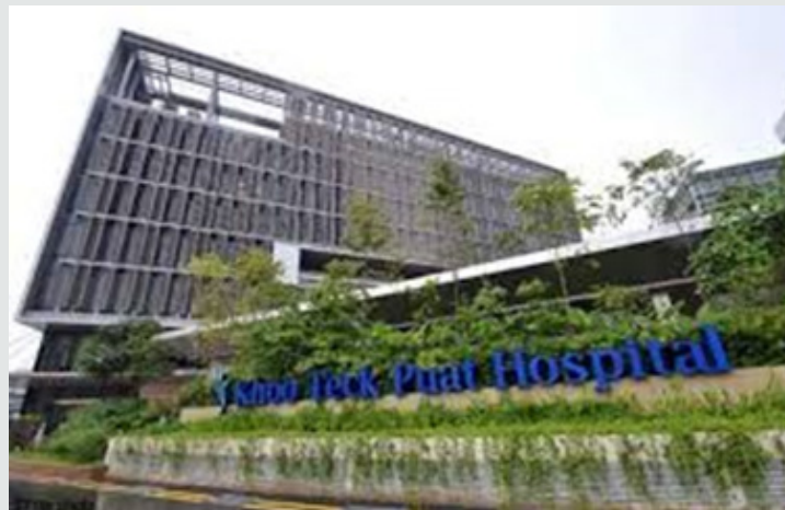
Figure 3: Khoo Teck Puat Hospital showcasing a hospital in a garden and a garden inside a hospital. (Source: Khoo Teck Puat Hospital. Image by Alexandria Health).
